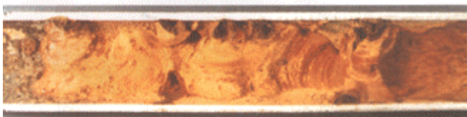
Pitting and hollows (Photo: CEBTP)
